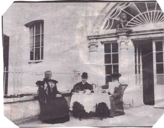
Imposing entrance to Vernon Mount as it appeared circa 1910. The house is currently (2011) in foreign ownership and is very dilapidated. Given its historical significance and grand design, efforts are being made to have the house taken into public ownership in order to have it restored to its former glory. 18
